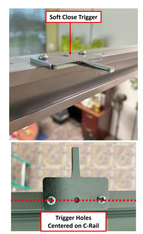
Attaching the Trigger:
